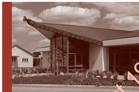
Tainui's Te Kauhanganui building at Ngapuna
